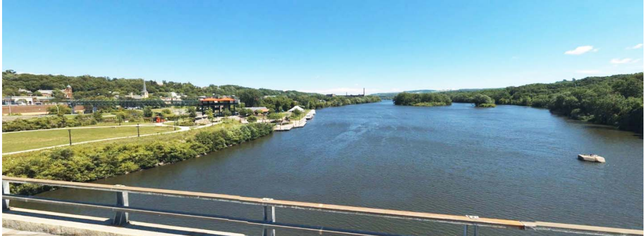
Inset 10. Mohawk River view east from Highway 30 bridge City of Amsterdam.
