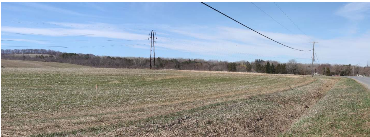
Inset 4. Pattersonville Road, Florida.
